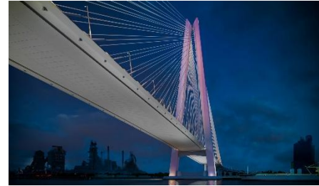
Gordie Howe International Bridge
